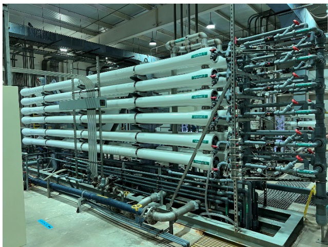
Reverse osmosis vessels at Reclamation's Water Quality Improvement Center in Yuma, AZ.
