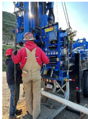
(Top) Project 21049 Monitoring while drilling
